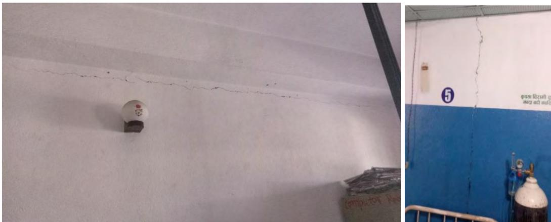
Figure 9: Cracks in walls
