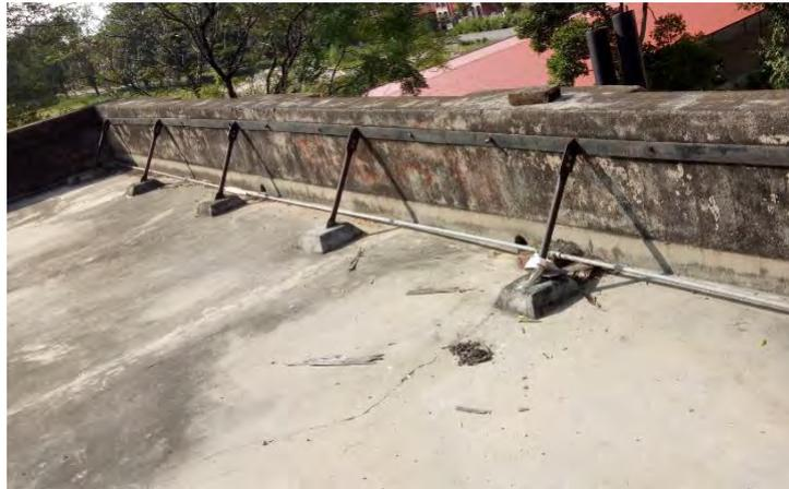
Figure 14: Parapet wall anchorage
