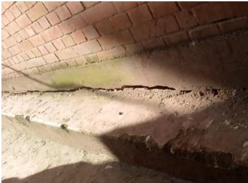
Figure 11: Settlement cracks in Maternity Block
