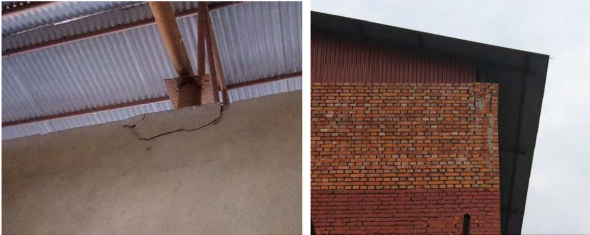
Figure 10: Cracks at truss and wall joints of Main Blocks
