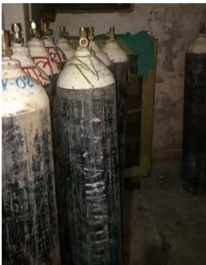
Figure 13: Oxygen Cylinder Kept Unbraced
